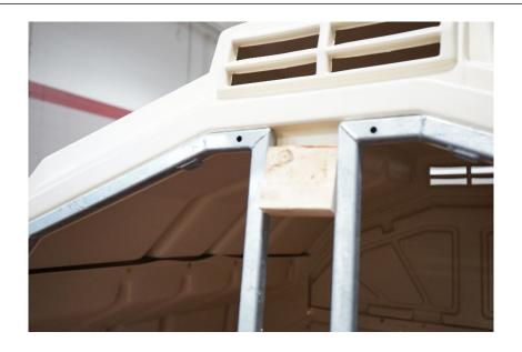
Once both front Frames are installed, the bottom of the Frames can be screwed down using the supplied lag screws and washers in the hardware kit.
