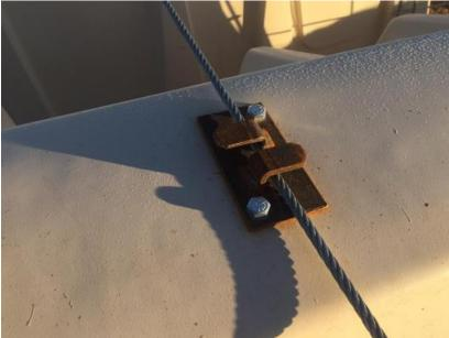
In areas with strong windstorms, calf raisers sometimes choose to secure hutches by attaching a latch similar to this to the top of the hutch and run a cable the length of the row of hutches, anchoring it at both ends.
